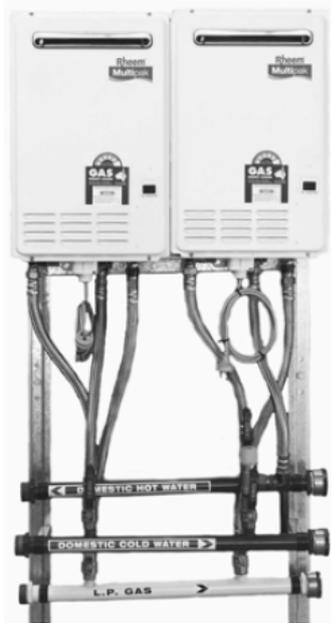
Figure 4-13: Typical Multipak setup (Rheem 2007)
