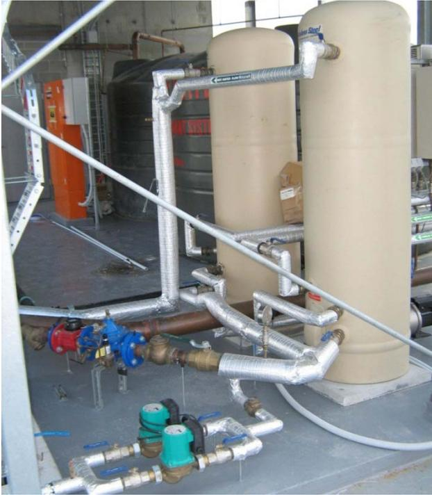
Figure 4-12: Heater and hot flow and return pipe tank connections in La Banque gas ring main plant
